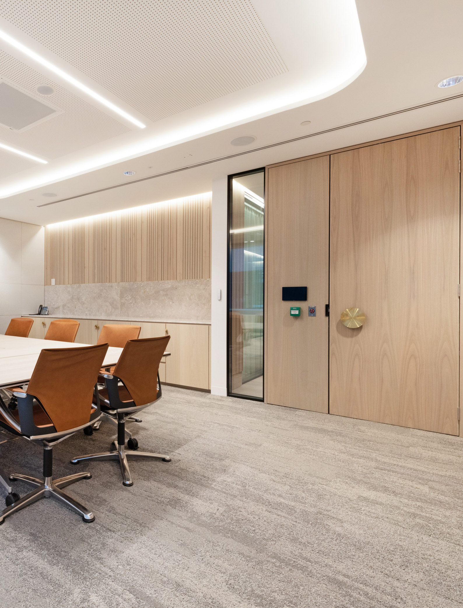
Ashurst Canberra. Design by Linear Designs. Featured: solid core & full glazed MDF doors with eucalypt veneer.
